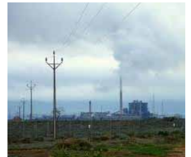
Port Augusta Power station
